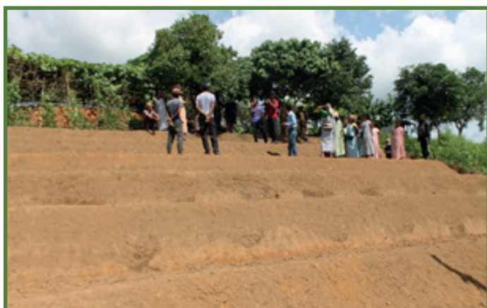
Newly constructed terraces
